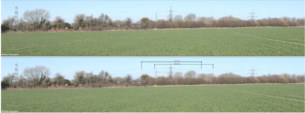
IMAGE 3. National Grid's Environmental Statement Appendix M, View 4a, which is from a viewpoint along Crooks Lane immediately to the west of our Clients' property, and is effectively the landscape they look onto and reveals the real dominance of the pylon infrastructure:
